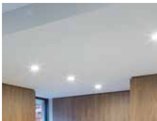
Led Lighting Internally
